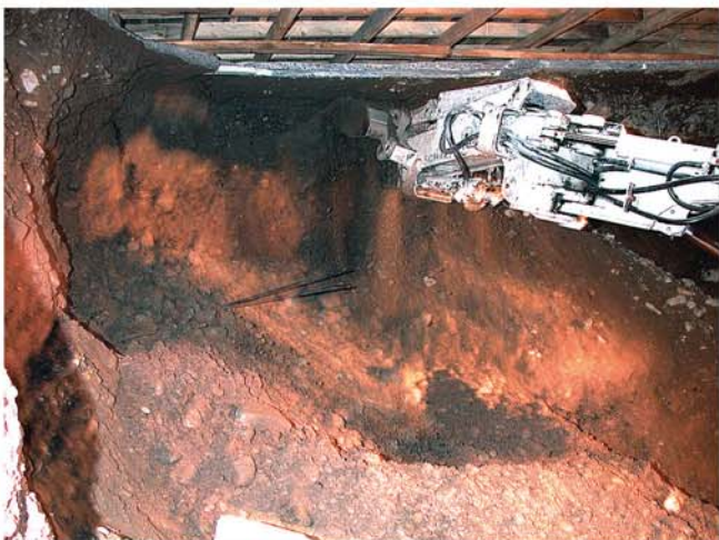
Accurate working, the roof must not be damaged
