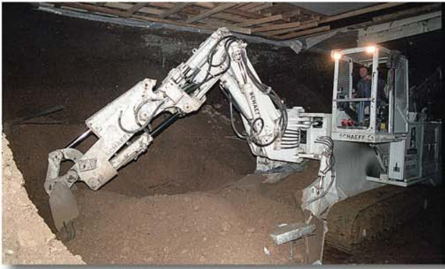
High loading capacity up to 5 m 3 /min
