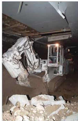
Loading of big blocks
