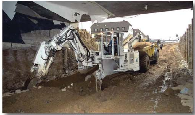
Invert cleaning works at the tunnel entrance portal
