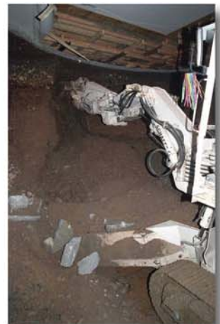
High efficiency excavation
