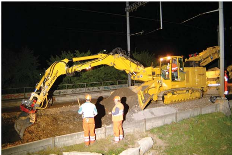
Reduced space requirement thanks to onboard conveyor
