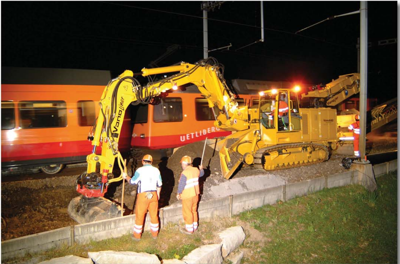
The ballast loading machine Schaeff model ITC 312 VL2 with jointed boom in loading position
