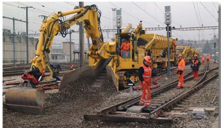
Reduced space requirement thanks to onboard conveyor
