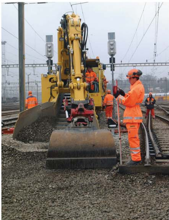
Acurate working thanks to the Roto-Tilt device
