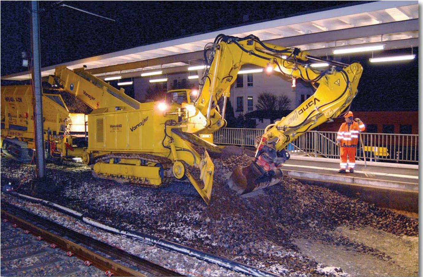
The ballast loading machine Schaeff model ITC 312 VL2 with jointed boom in loading position
