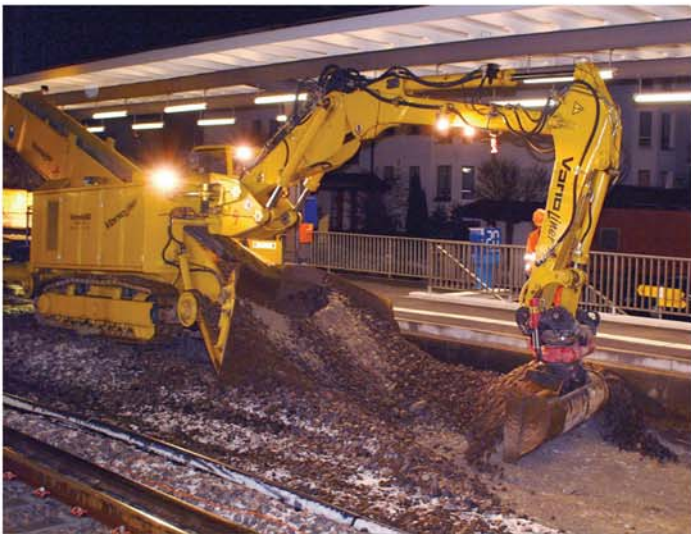
Reduced space requirement thanks to onboard conveyor
