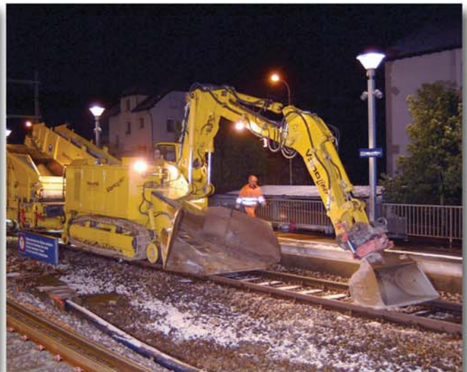
Accurate working thanks to the Roto-Tilt device
