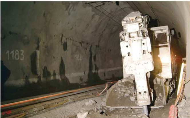
The Heading Machine model ITC 320 while lowering the invert with the hammer V45
