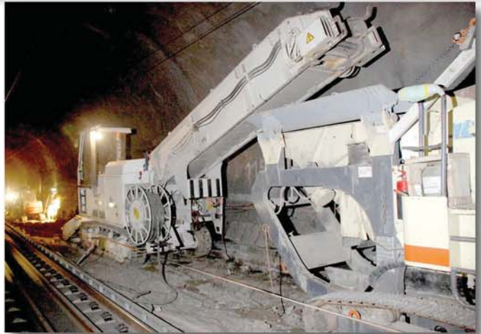
The Tunnel Heading Machine ITC 320 loading in a crusher
