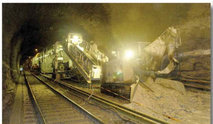
The Tunnel Loading Machine ITC 112 E4 loading in a conveyor
