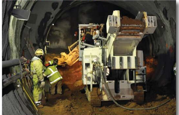
Fig. 6: Excavating the left bench
