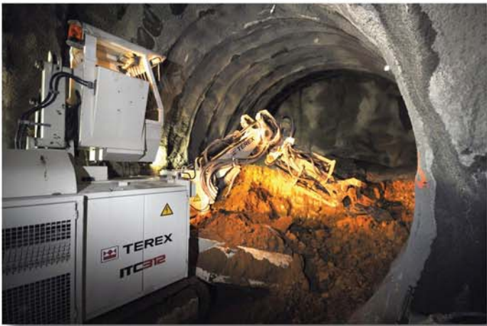
Fig. 3 Excavating the right bench
