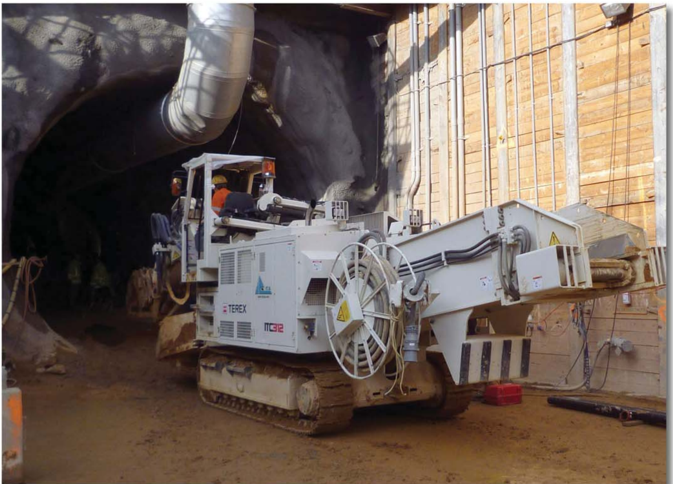
Fig. 1: ITC 312 at the right portal entrance
