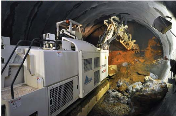
Fig. 7: Excavating the middle bench
