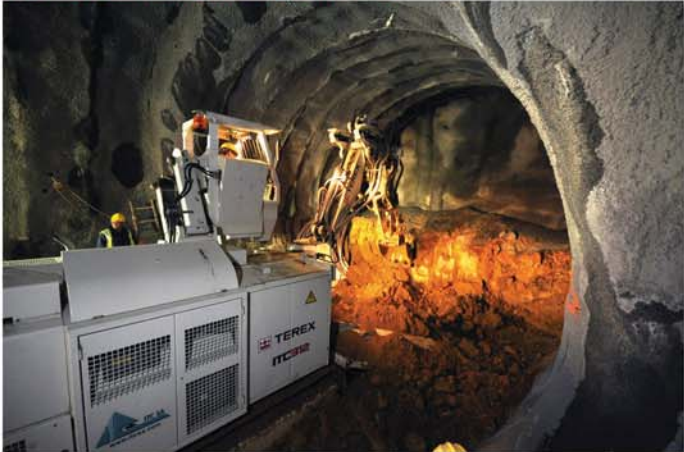
Fig. 5: Excavating the middle bench
