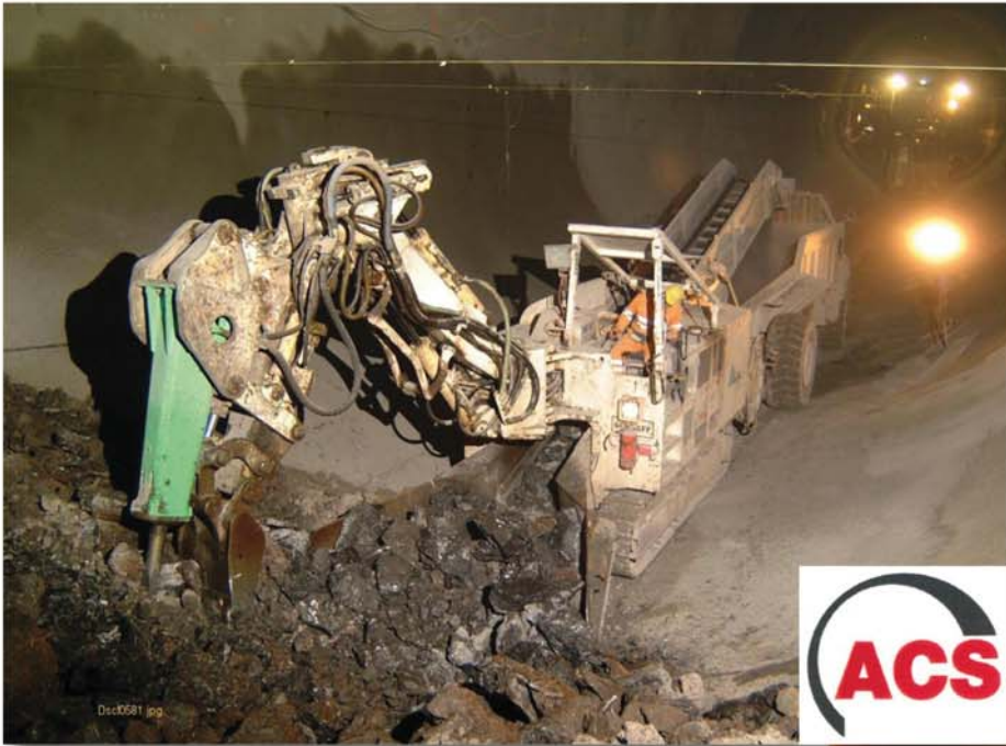
Fig. 7: At bench excavation in the West
