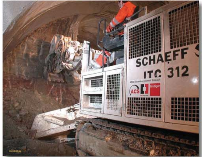
Fig. 12: At the vault extension in the West
