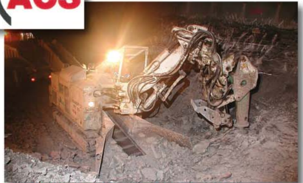
Fig. 10: At bench excavation in the West
