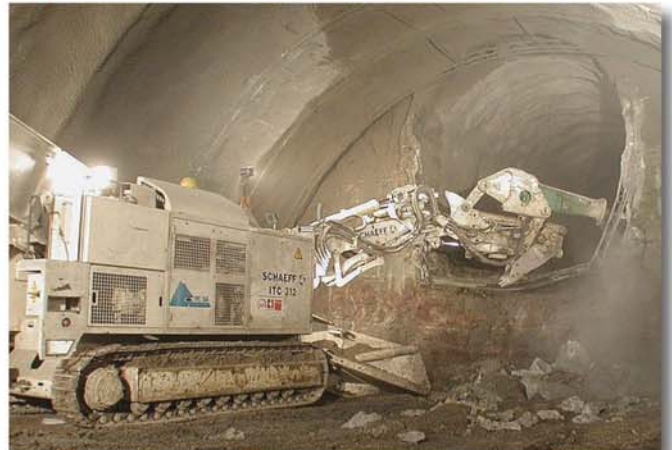
Fig. 13: Expansion of the pilot tunnel in the West
