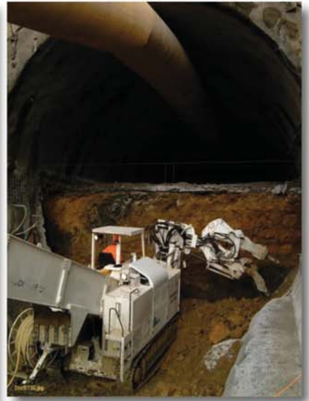
Fig. 8: At bench excavation in the East
