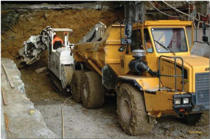
Fig. 9: Loading onto 25 t articulated dump truck
