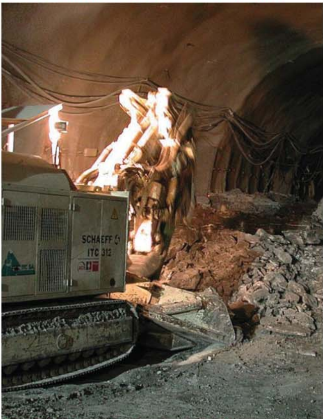
Fig. 11: At the vault extension in the West
