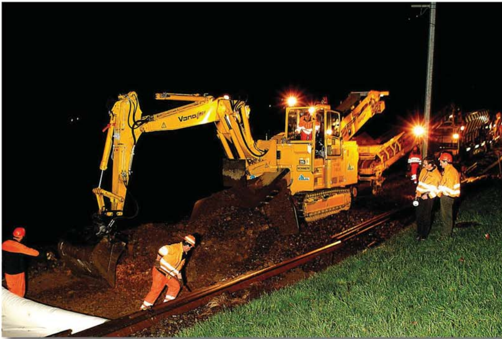
Pict. 7: Working between slope and road on 1:20 gradient BALLAST
