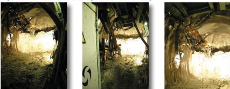
Fig. 13 – 15: Drilling gear on the GTA Tunnelling Gantry
