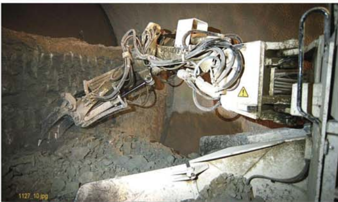
Fig. 12: ITC when excavating the hard marl clay
