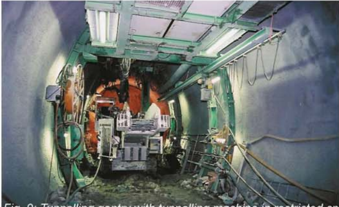
Fig. 9: Tunnelling gantry with tunnelling machine in restricted space
