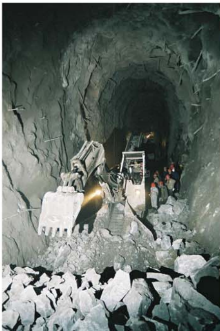
Picture 11: Mucking in the main tunnel
