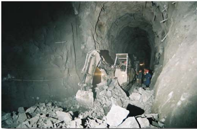
Picture 7: Mucking in the main tunnel
