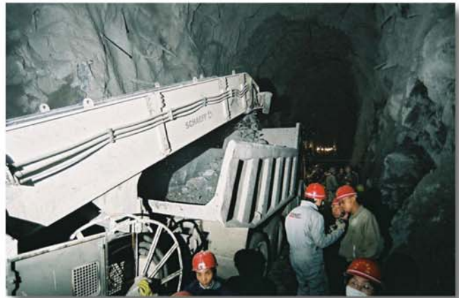
Picture 8: Loading onto Isuzu 20t dump trucks
