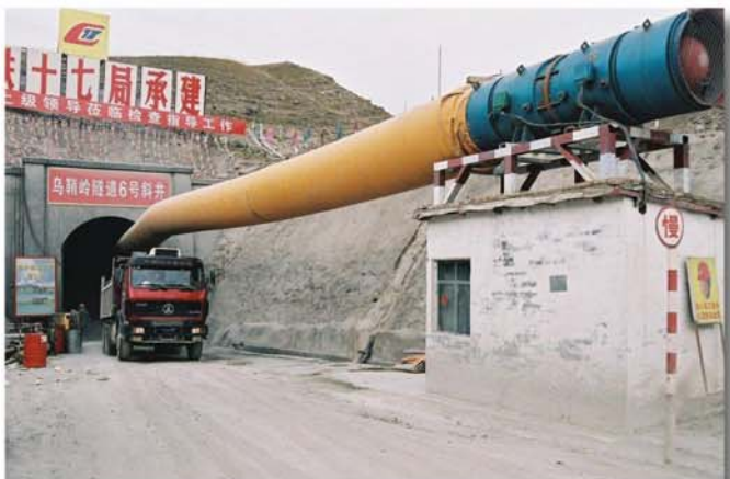
Picture 10: Portal of the access tunnel ..
