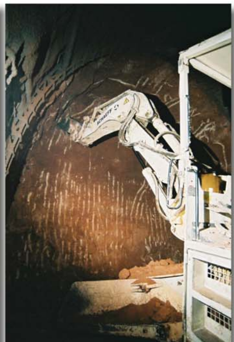
Picture 13: Access tunnel driven in soft rock
