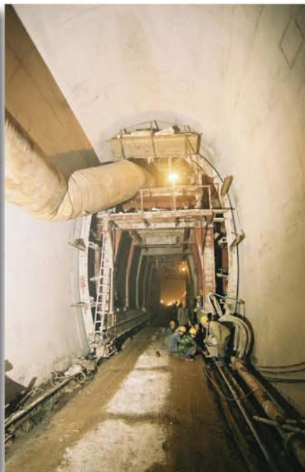
Picture 12: Shutter in the main tunnel
