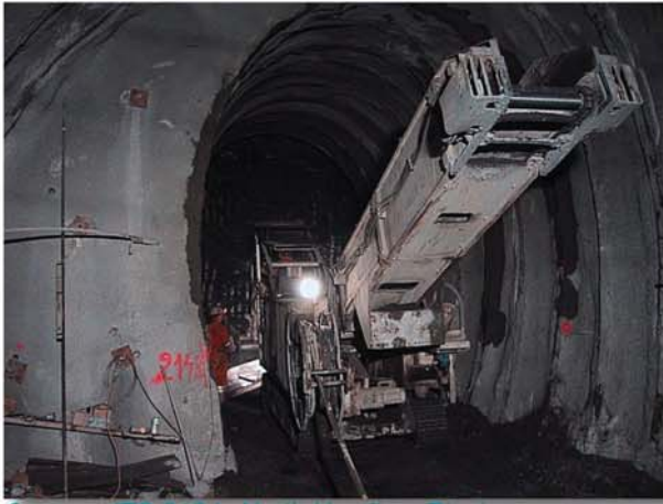
6: ITC 312 in North Heading, Ripping
