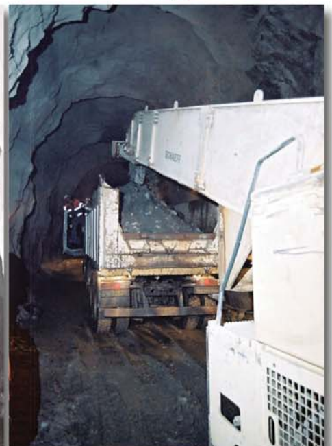
Pict. 6: Conveyor extension to fill the truck
