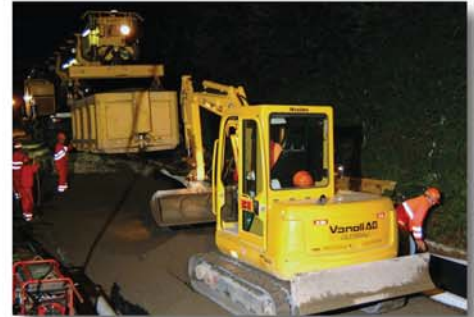
Bringing in the new material by crane
