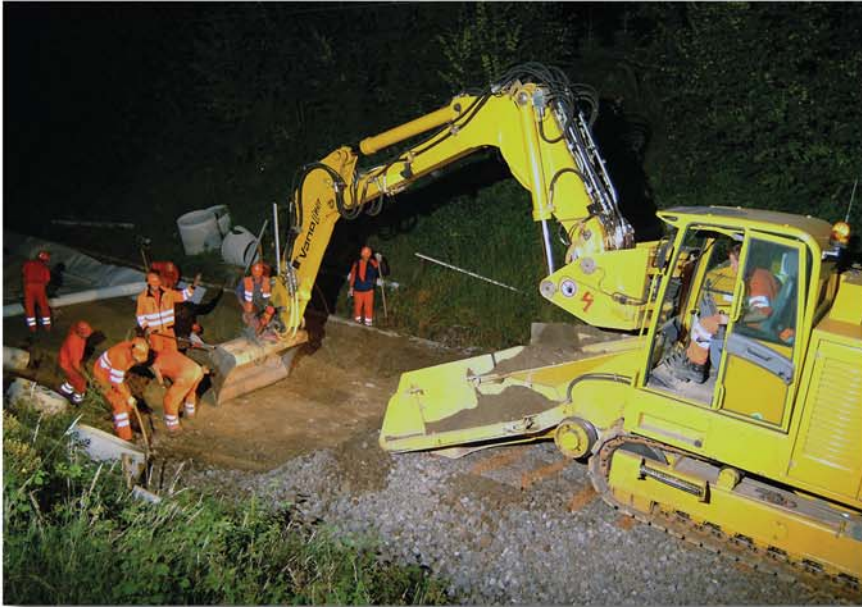
Exact levelling thanks to laser control
