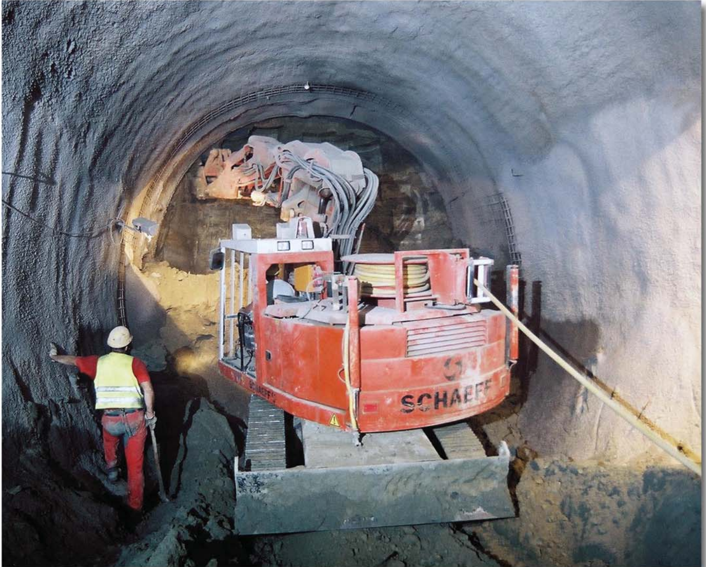
Heading in typical subway cross-section in Munich
