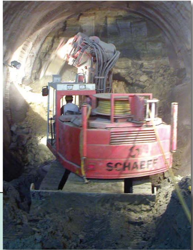
Acurate excavation thanks to swivel dipper stick ->
