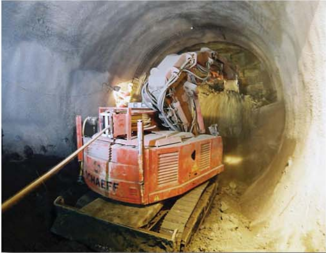
Excavation in the fore polling heading
