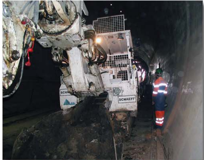
The compact Tunnel Heading Machine Schaeff model ITC 112 M4
