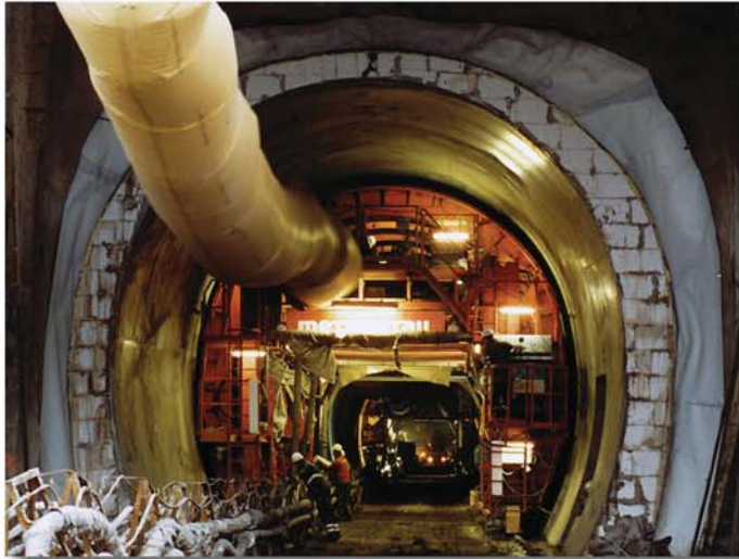
Schutter for the secondary lining
