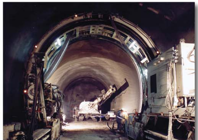
The saw cutting machine and the Jet drilling machine
