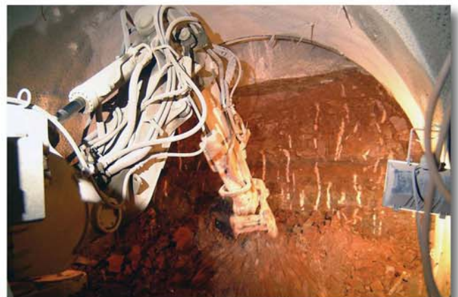
Excavation of the cross-section
