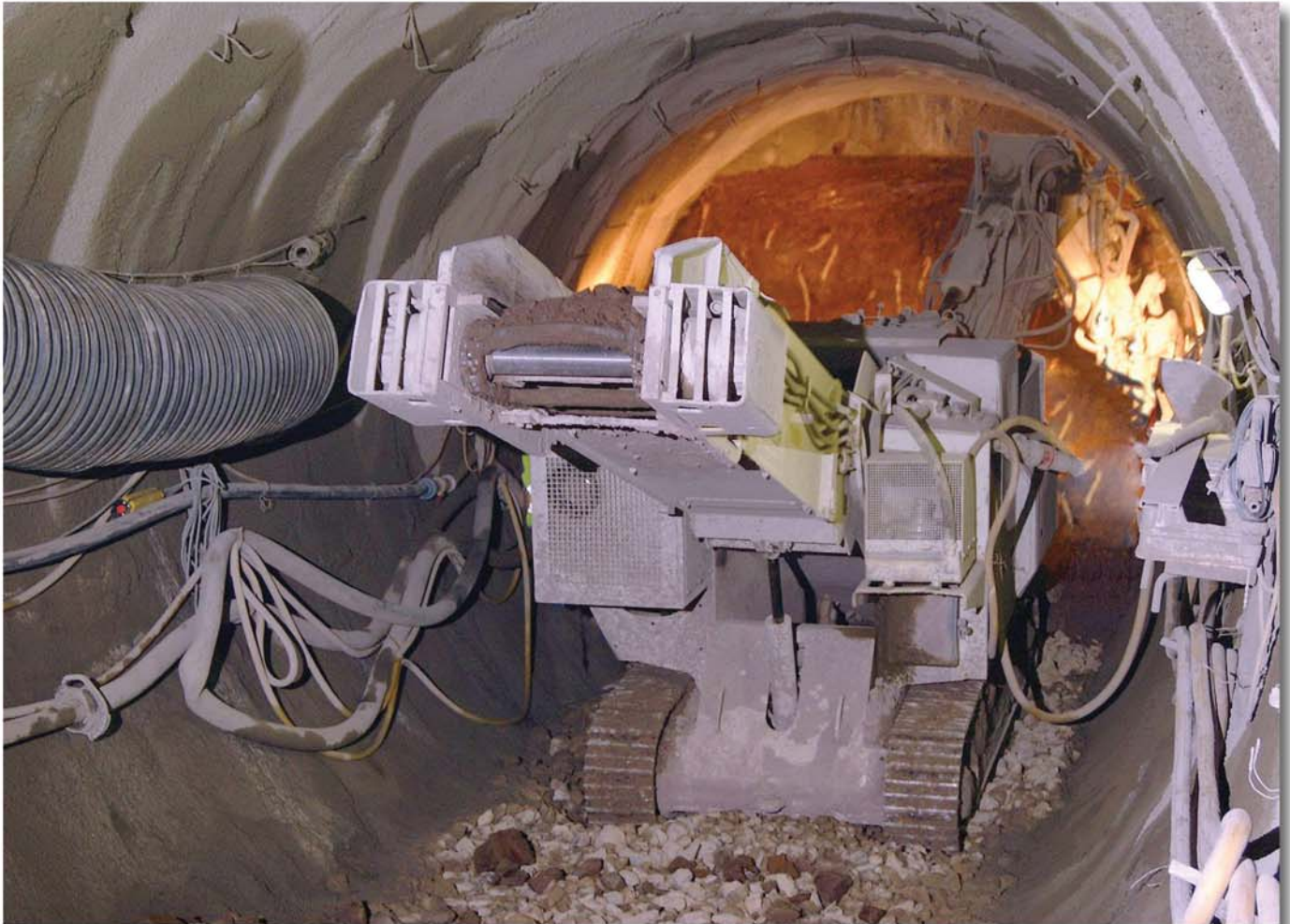
The tunnel heading machine Schaeff model ITC 112 E3 in excavating position
