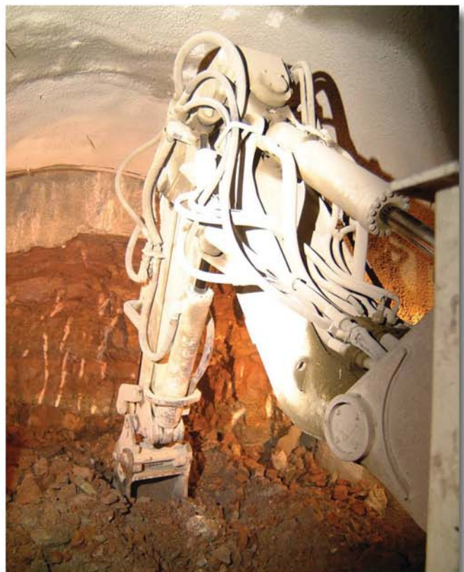
Excavation of the bench
