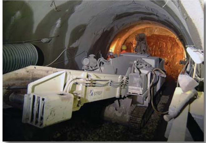
Tunnel Heading machine
