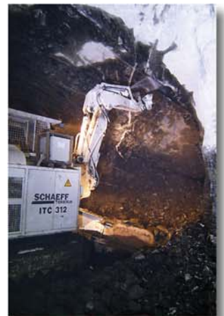
Scaling the loosed blocks
