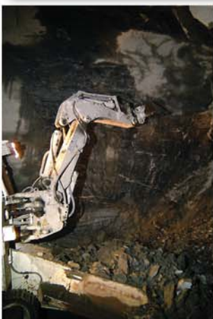
The loading machine ITC 312 while scaling
