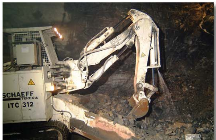
The loading machine ITC 312 while mucking at high speed
