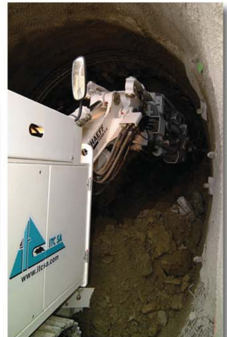
The Tunnel Heading Machine excavating the soft material
