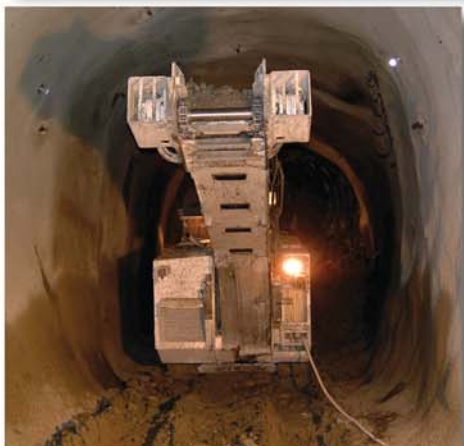
Rear view in the narrow tunnel
