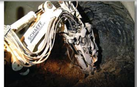
Mucking out the blasted material
