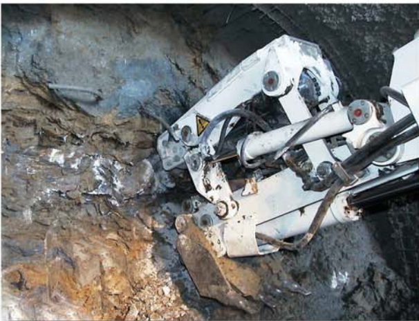
The Heading Machine Schaeff model ITC 120 while excavating with the hammer
