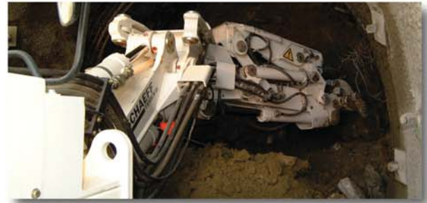
Acurate excavation thanks to the tilt and sviwel console
