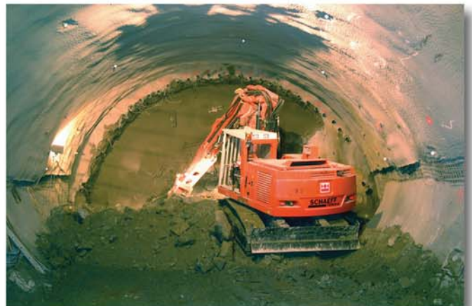
The Tunnel excavator model TE 200 climbing on the muck pile to excavate the crown
