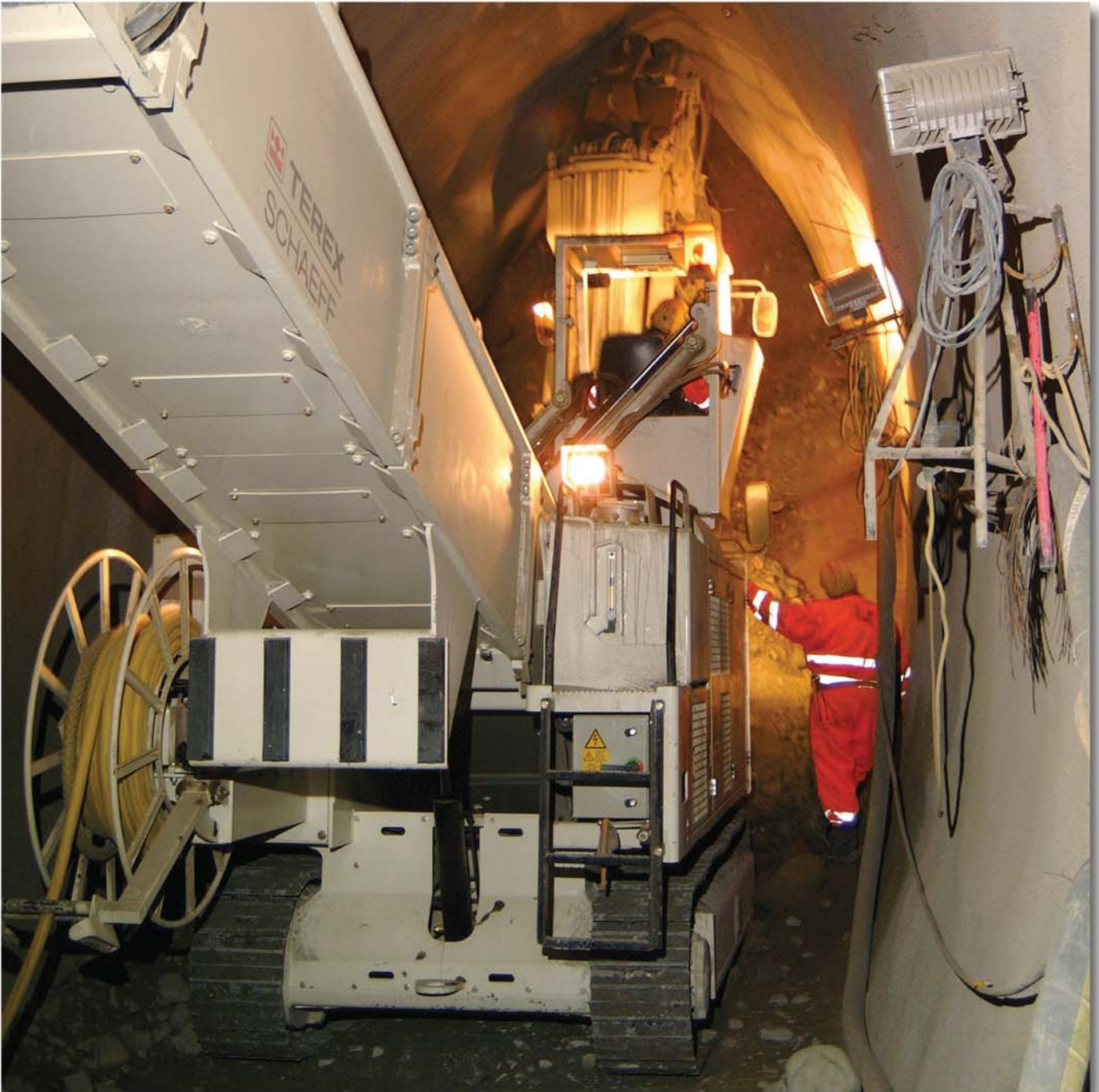
The Tunnel Heading Machine Schaeff model ITC 312 N1 in excavation position under the concrete prevaults
