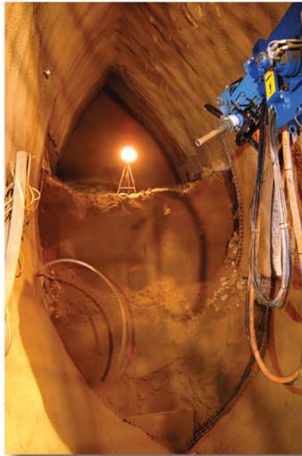
The compact Tunnel Heading Machine Schaeff model ITC 112 M4
