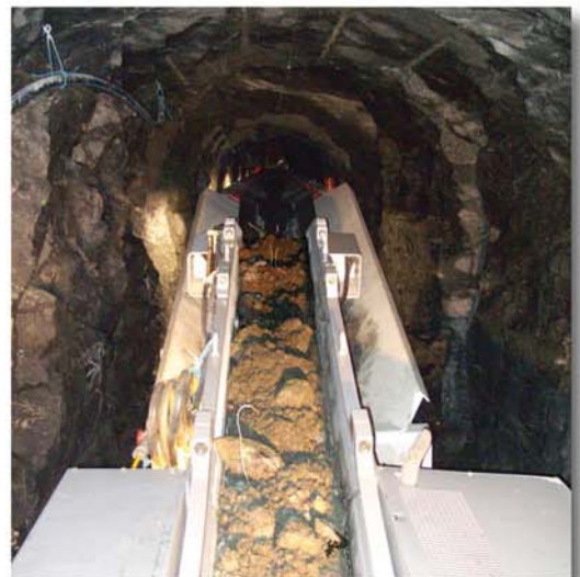
Continuous loading of the blasted material
