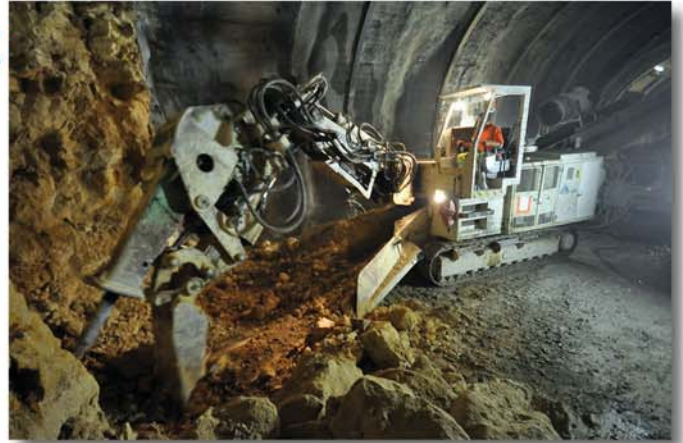
Fig. 9: ITC 312 by sole cleaning
