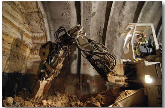
Fig. 7: ITC 312 with swivel cabin
