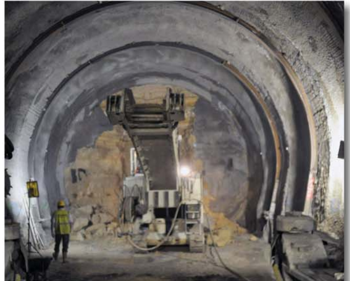
Fig. 13: Heading in the tunnel
