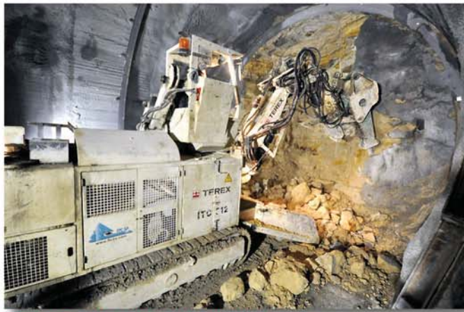
Fig. 6: Rock breaking in the hard clay
