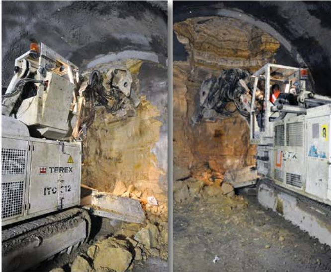
Fig. 12: Swivel cabin right respective left
