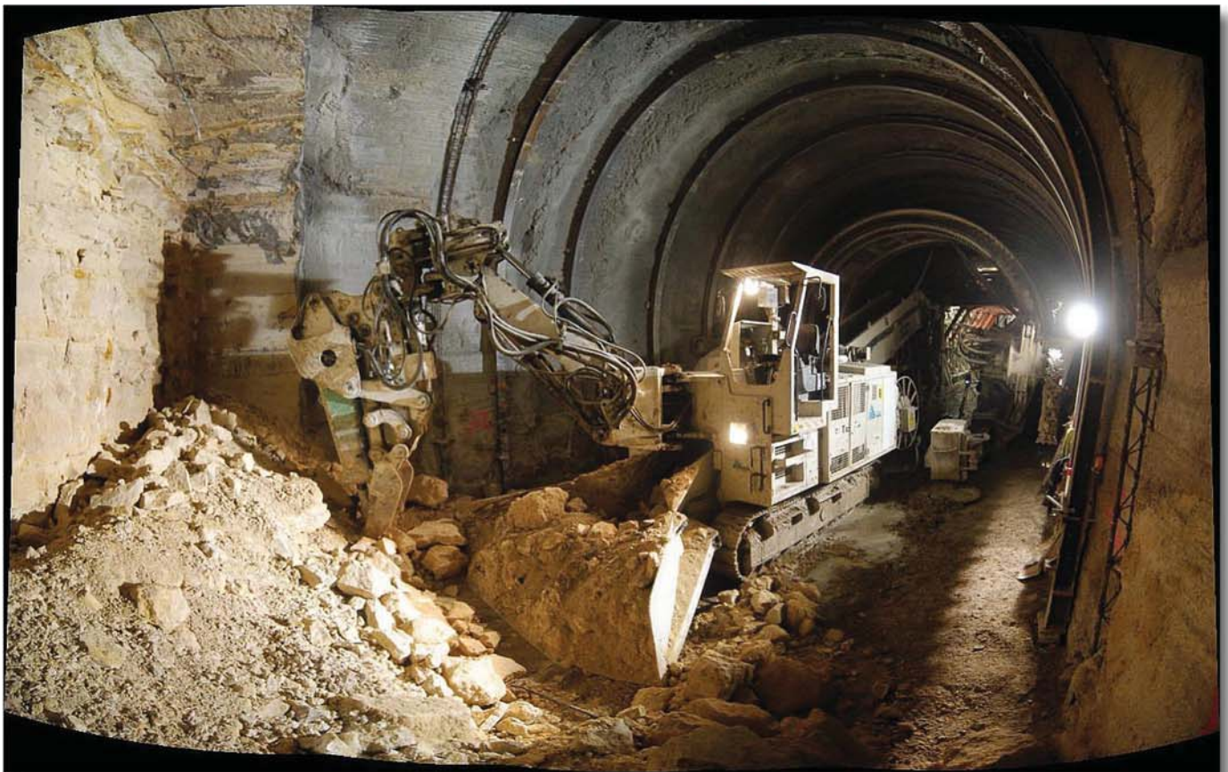
Fig. 1 : ITC 312H6 in the clay and ballast of Paris
