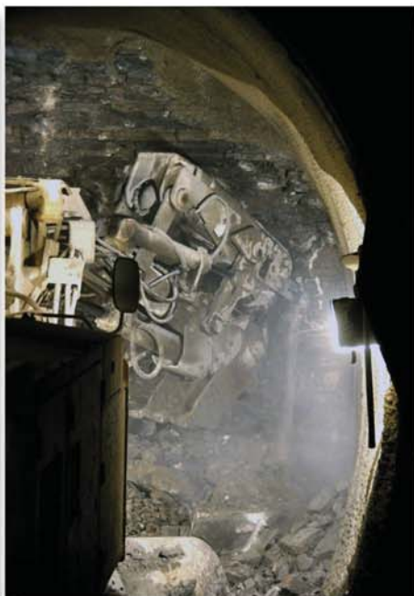
Fig. 5: rock breaking with hammer
