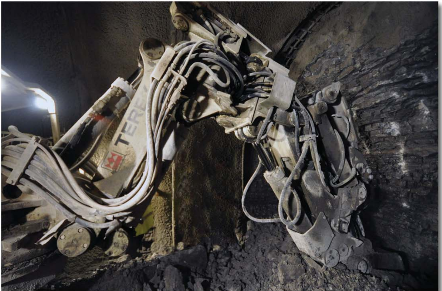
Fig. 1: ITC 120 F2 during Tunnel Heading
