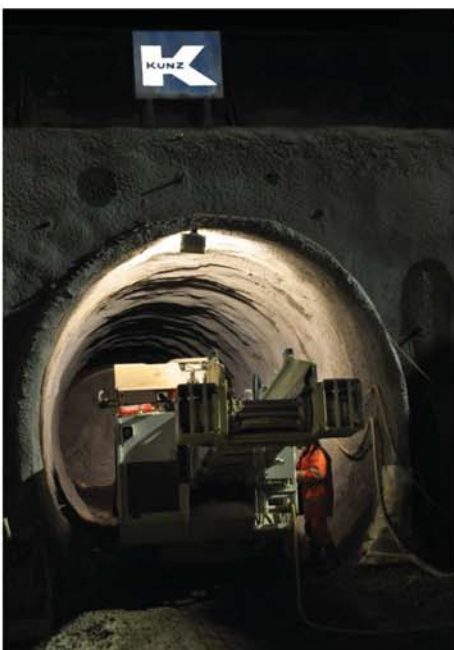
Fig. 8: ITC 120 at the tunnel entry
