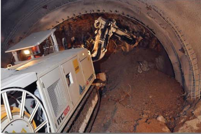
Fig. 8: Heading of the expansion (niche)
