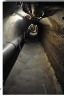
Fig. 3: Tunnel with ventilation
