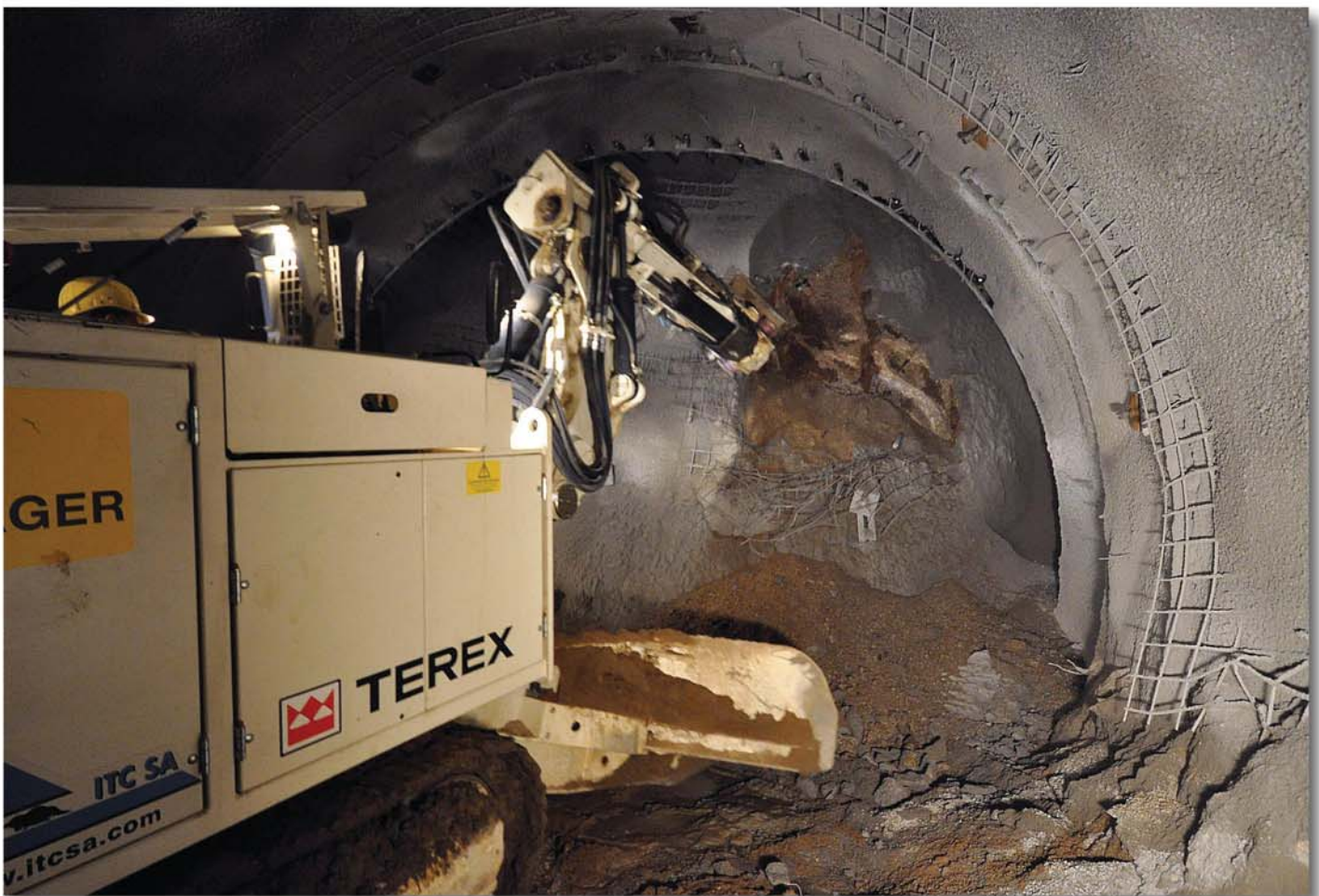
Fig. 1: ITC 120F3 during Tunnel Heading expansion
