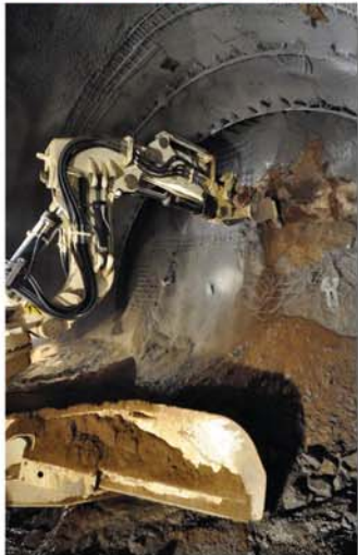
Fig. 12: Secured heading face
