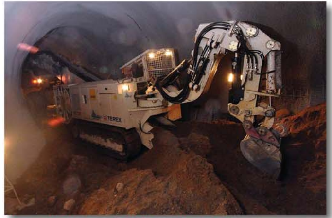
Fig. 7: ITC 120 while loading the debris
