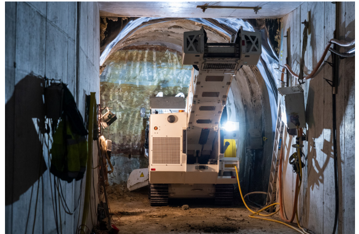
The 14.5m 2 section is narrow, but the ITC125 will work through it without any problems.
