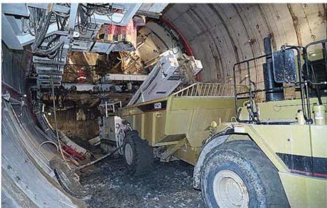
Loading onto 25t articulated dump truck
