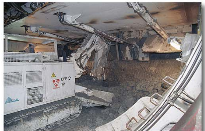
Loading also the excavation of the stationary excavator
