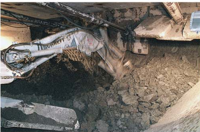
Excavation at the lower level of the shield
