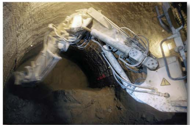
Excavation of the fore polling top heading
