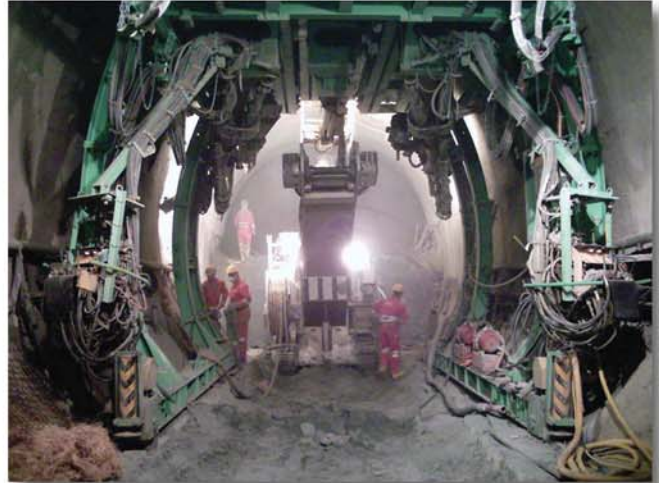
Tunnel Heading Portal for drilling and ramming purposes
