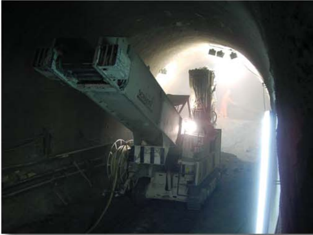
Rear view of the machine while shotcreting
