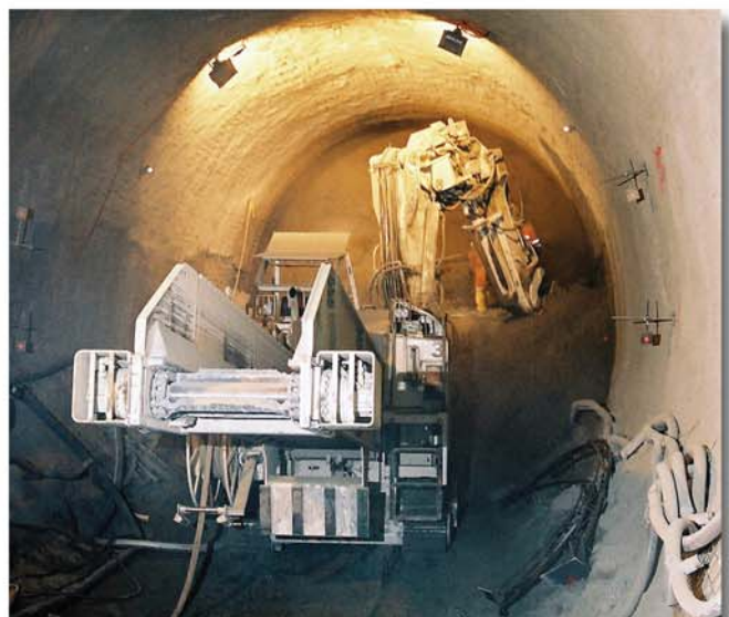
Excavation of the bench
