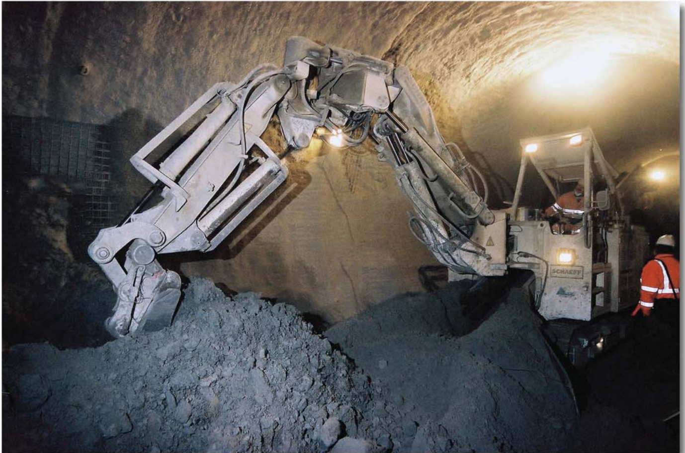
The tunnel heading machine Schaeff model ITC 312 N1 in loading position
