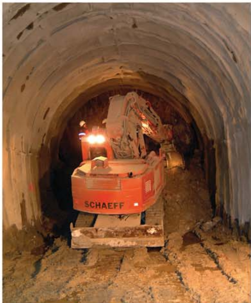
The Tunnel Excavator excavating the lifters
