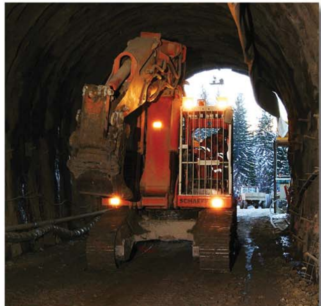
The Tunnel Excavator on its way to the face
