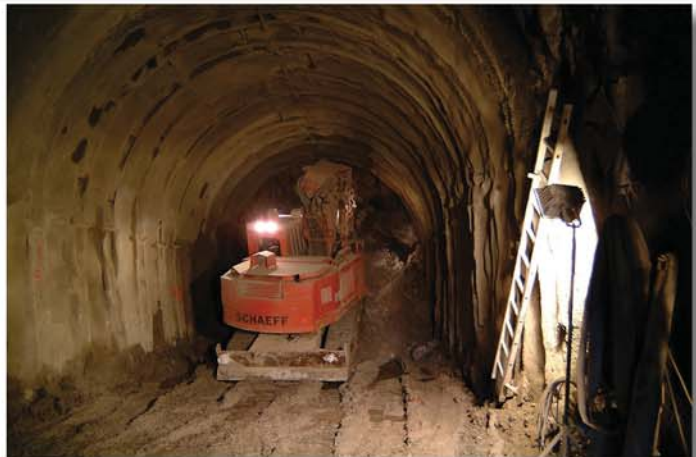
The Tunnel Excavator excavating the central bench
