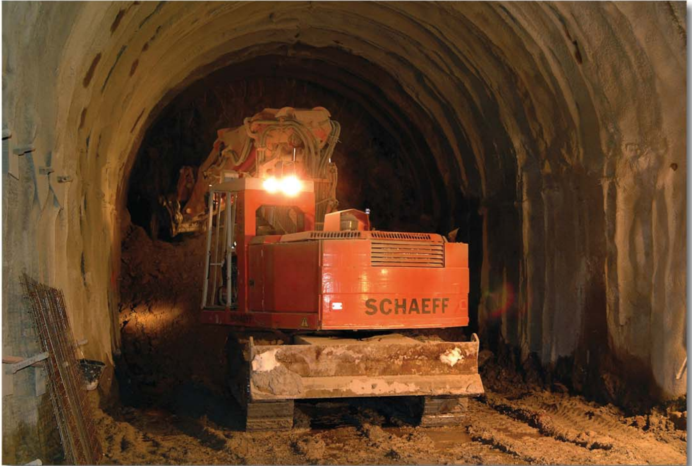
The Tunnel excavator model TE 200 in the 37 m 2 cross-section, crown height 6 m
