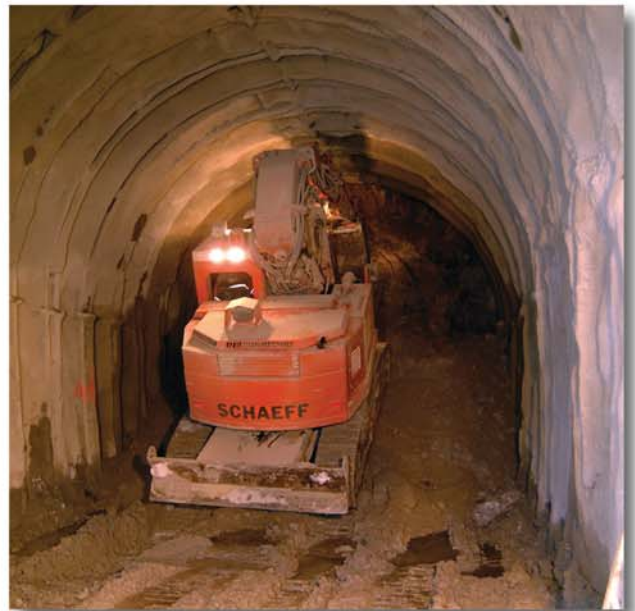
The Tunnel excavator model TE 200 climbing on the muck pile to excavate the crown
