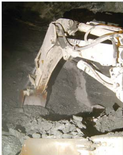
The Superloader ITC 312SL cleaning the invert
