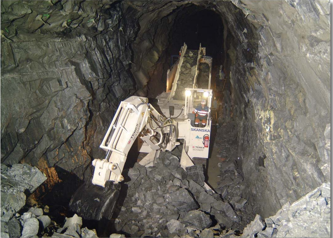
The Superloader Schaeff model ITC 312SL in loading position
